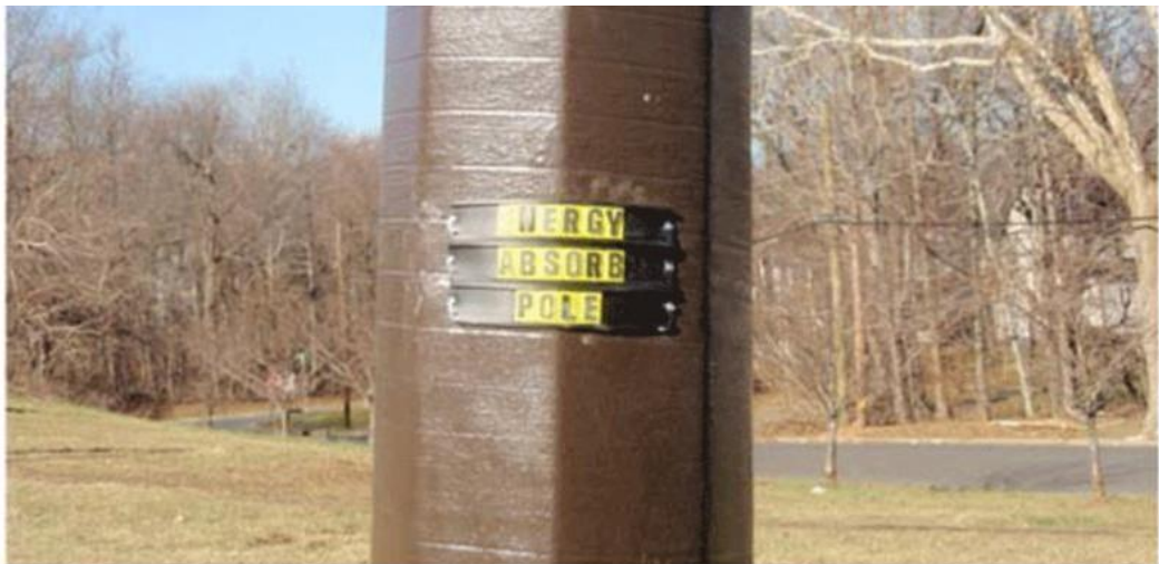
Figure H-1. Photo. A close-up of the energy absorbing utility poles used as a part of NJDOT's pilot project.
