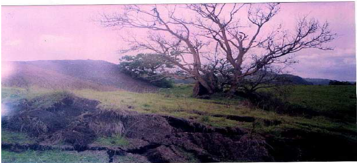
Fig.3.4. Damage of the tree and the surrounding land caused by the mass slide of the spoil
