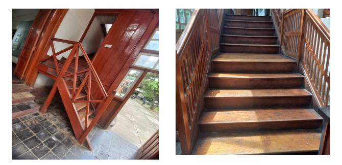
From the above pictures, we can see that the interior stair is not accessible and hard to walk because of long steps and inaccessible encounter which blocks communication for wheelchair and crunch users.
