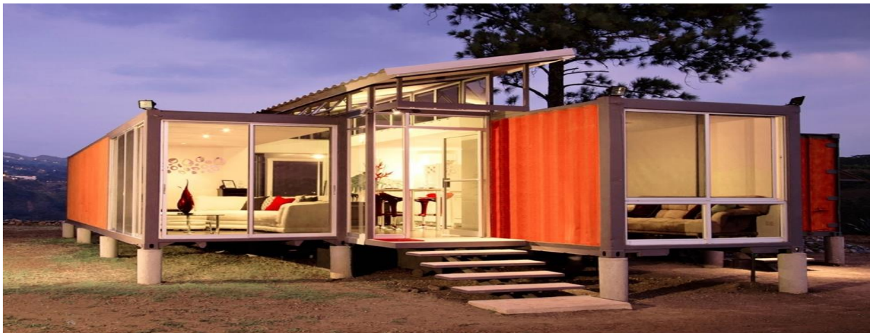
Figure 2. 2 Shipping Container Home
