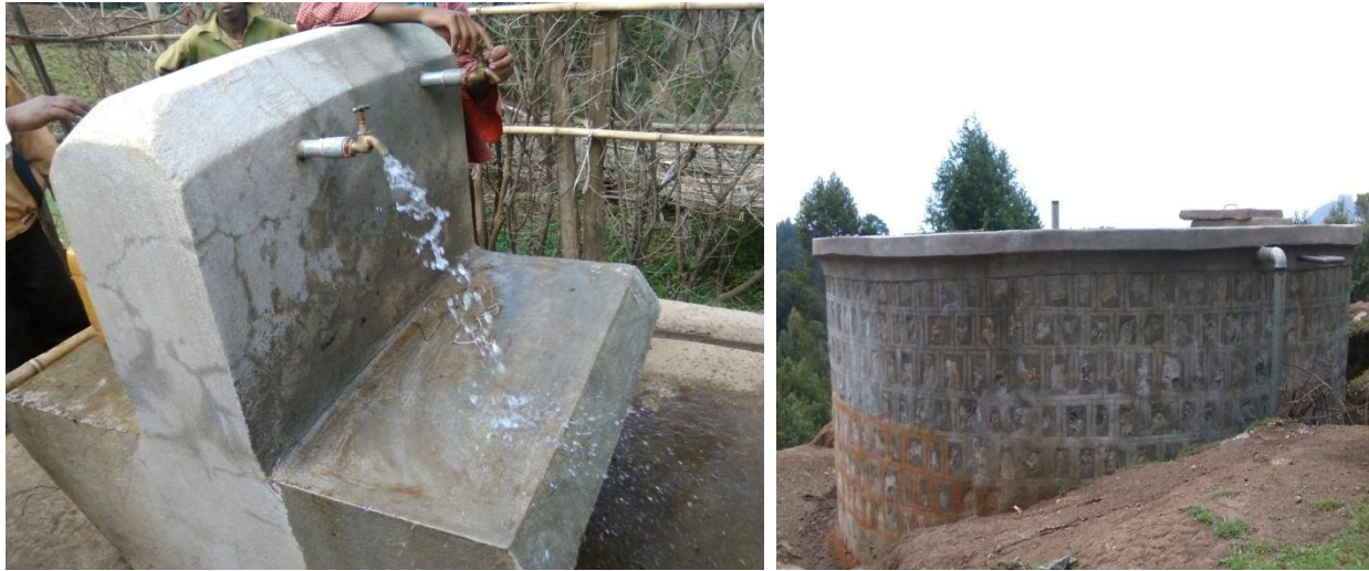
Figure 13, Water point and reservoir established by the project
