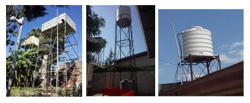
Figure: 4. 6 Common Ways of Placing House Hold Water Storage Tanks.
