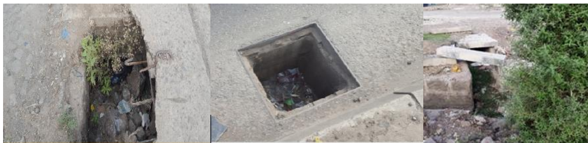
Figure 6: Pictures showing open drainages in some areas of sampled kebeles 01/02, 02/03 and 04/05 of Nefas-silk Lafto sub-city, Addis Ababa, April 2017
