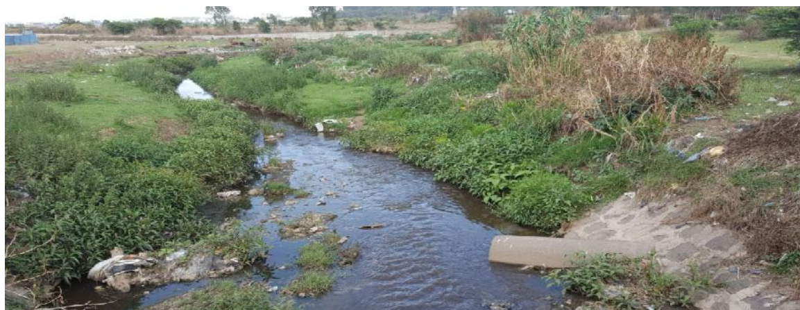
Figure 9: A river without a buffer zone (source: Field survey April, 2017)
