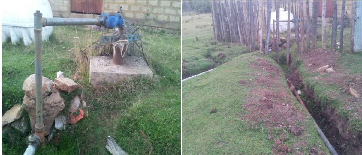
Plate 1: Dinkula town's borehole water scheme with two pipeline distributors, Endegagn Woreda
